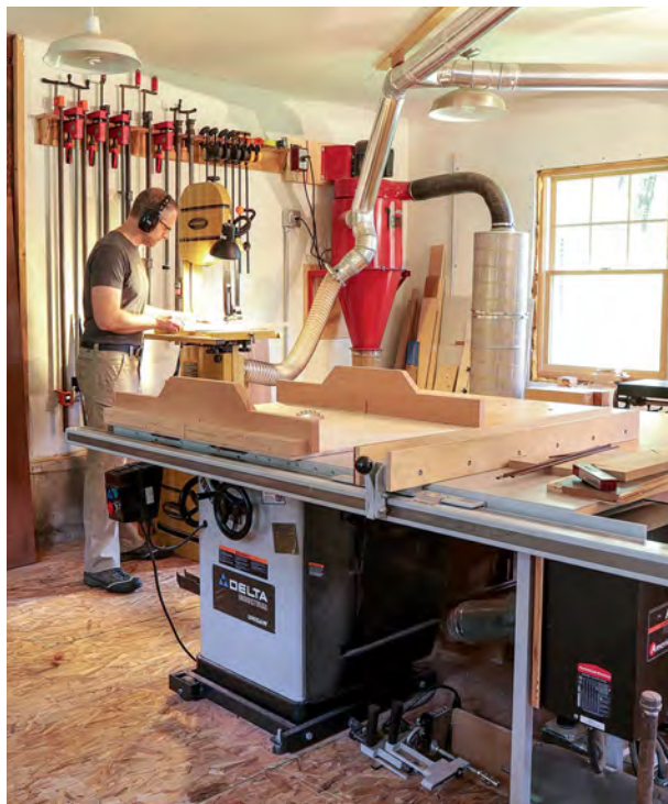
Collection in the corner. With the big machines clustered near the dust collector, only a small amount of ducting was required to serve the tablesaw, planer, jointer, and bandsaw.
