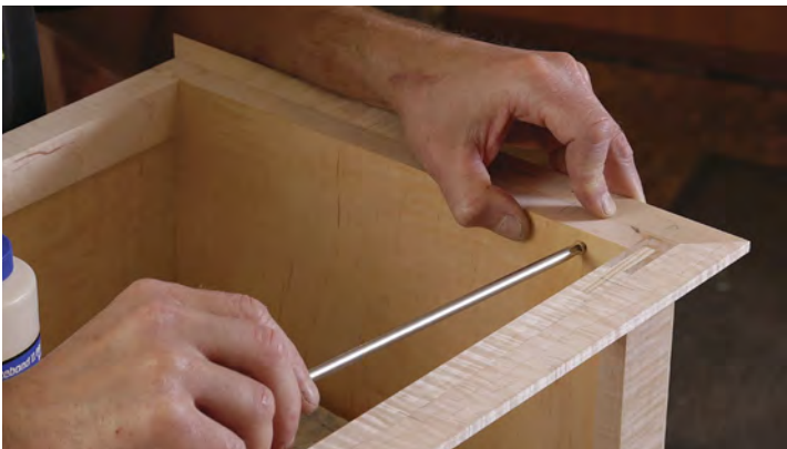
Fixed at the front. The side molding is screwed and glued at the front end, but not at the back, where it is held tight to the case by the cleat.
